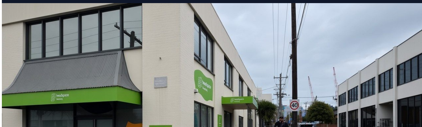
Facade restoration, Headspace, 105 Yarra Street, Geelong
